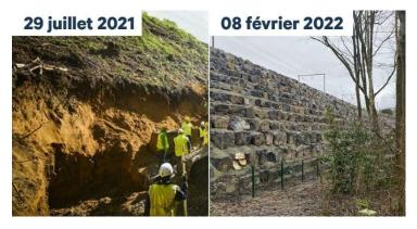
A total of 10,000 m³ of soil had to be removed as it threatened the stability of the tracks. Our teams thus managed to secure the zone to ensure continuity of train traffic.
