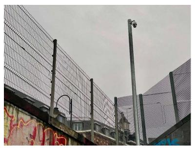
This device is composed of eight columns integrating infrared beams and connected fences fitted with two 360° cameras. This investment amounted to 370,000 euros. In the long term, this device is also due to be installed at four other key points on the Belgian railway network.
